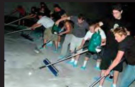
Sizing coating crew
